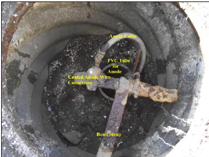
Typical soil side anode installation
