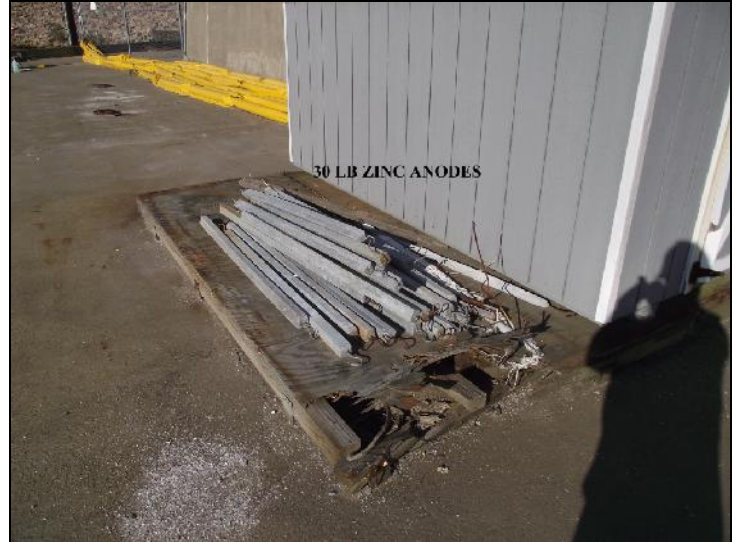
Unused zinc anodes for replacement
