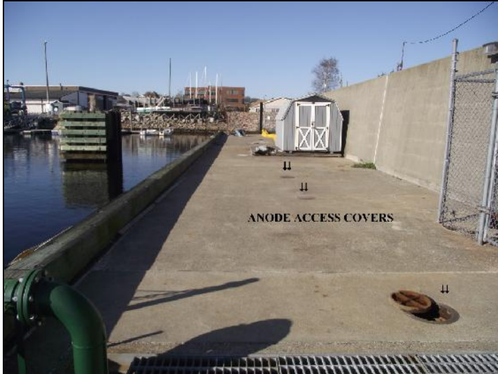
West end of dock and sheet pile
