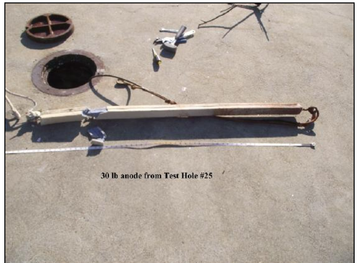
Zinc anode pulled from station 25
