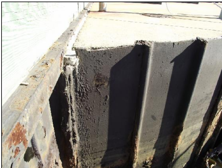
Typical sheet pile condition at top
