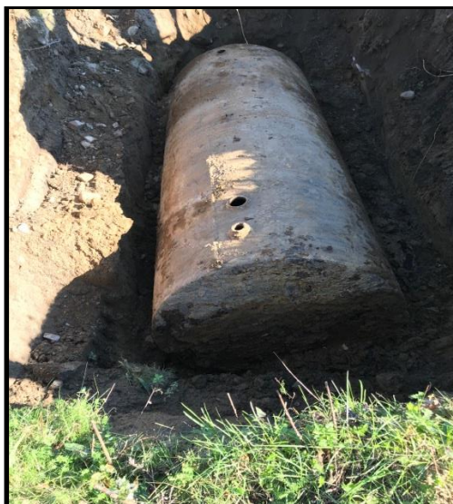
Underground Storage Tank Removal
